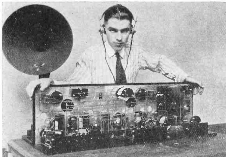
José Velasco and a general view of the rear of his receiver. Note the aluminum shield.
